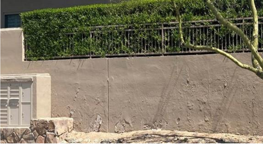
Figure 1 Water damaged wall.
